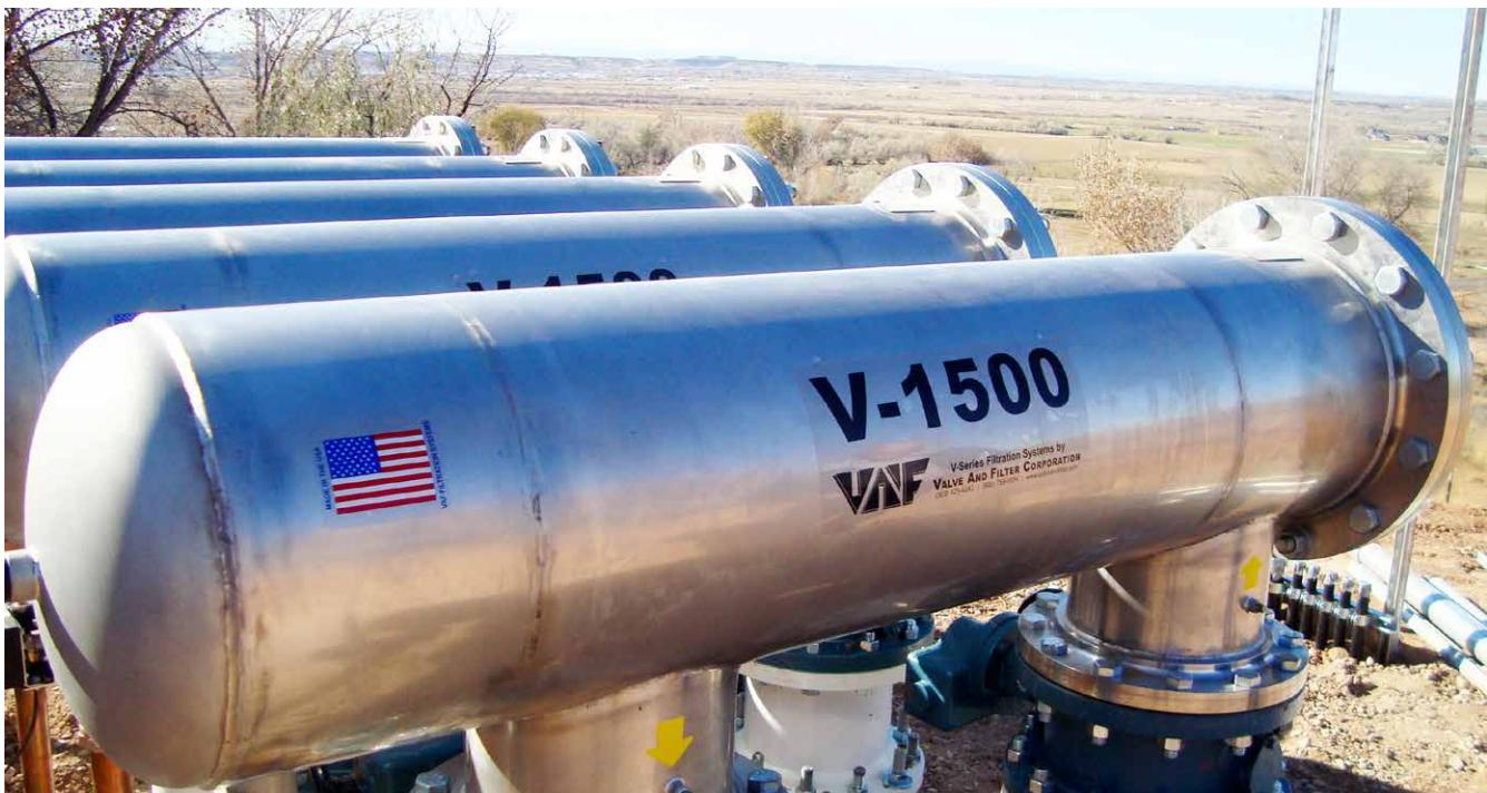
Five tanks used to filter sand and debris out of water for use by a rural community. (USACE photo by Scott Stoddard)
