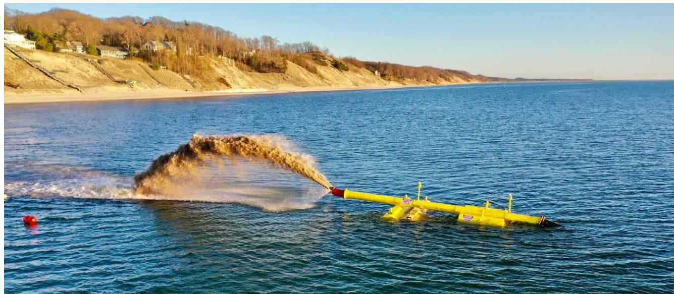
Maintenance dredging operations to place sediment in a nearshore area. (Photo courtesy of USACE)
